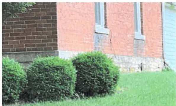
Example of original stone foundation
